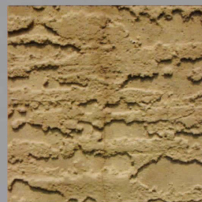
Bridges Hairline Cracks
